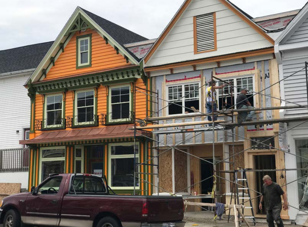
YARMOUTH FACADE PROGRAM
